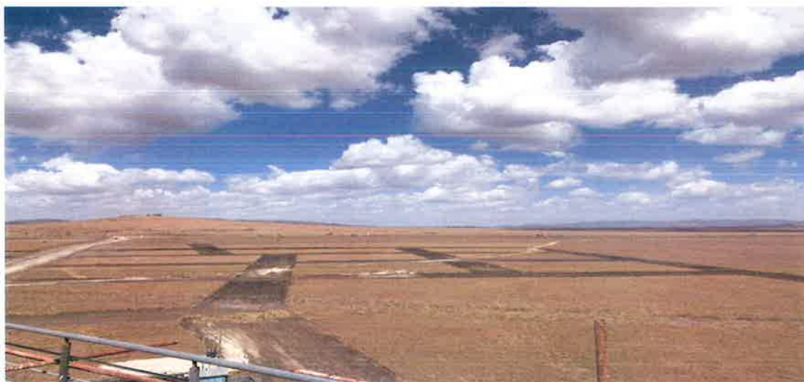
Aerial view of Access road under construction
