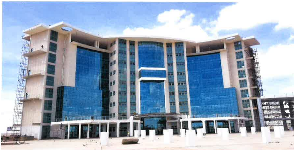
External view of Konza complex
